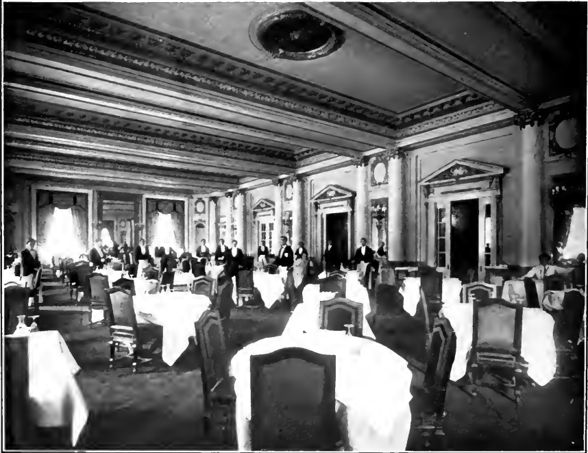
THE PALM-ROOM AND THE RESTAURANT OF THE HOTEL BELVIDERE. Baltimore, Md. Parker & Thomas, Architects.
